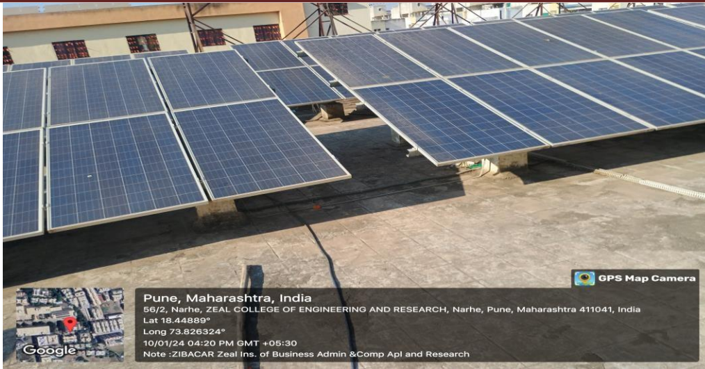
( 120KW Net metering solar PV Roof top system in the Campus)
