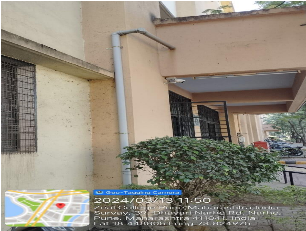
Image-7.1.4 (1b) -Rain Water Harvesting System
