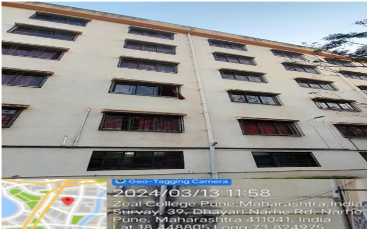
Image-7.1.4 (1a) -Rain Water Harvesting System
