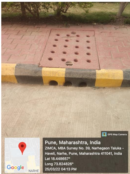
Image-7.1.3.2-Water Drainage Chamber at ZES Campus
